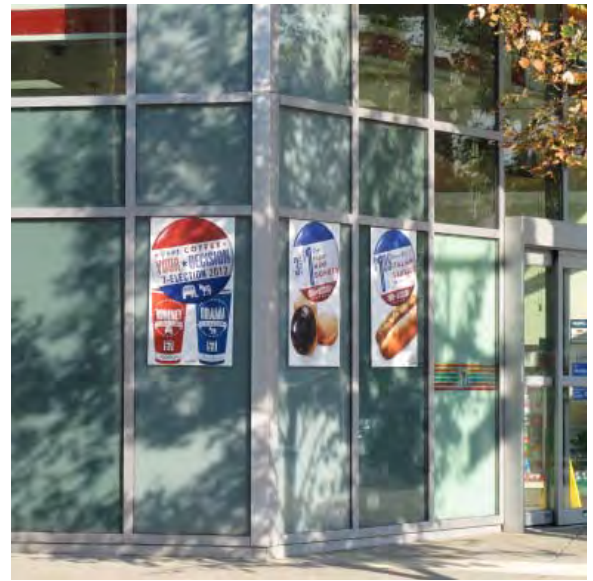
Portland & Main St., Cambridge, MA 7-11 windows obscured by frosting and signs
