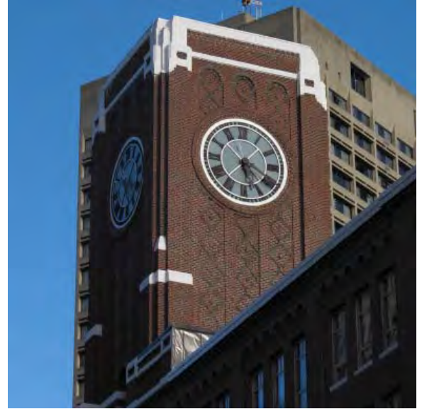
238 Main St., Cambridge, MA Kendall Square Building clock tower
