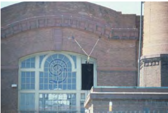
Bishop St., Framingham, MA Power plant, Dennison Mfg.
