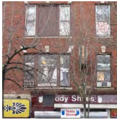
Massachusetts Avenue, Cambridge, MA signs in 2d and 3d story windows
