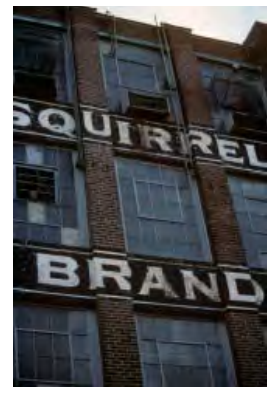
Boardman St., Cambridge, MA Squirrel Brand candy factory: the sign panels ignore columns, but respect windows and spandrels.
