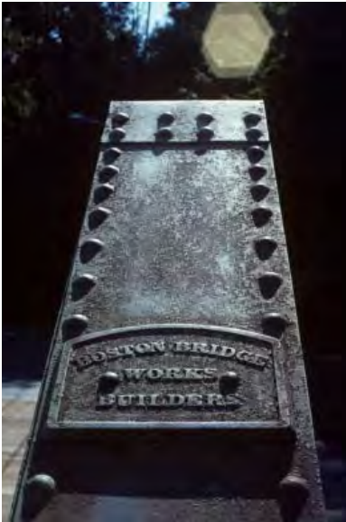
Albion, RI bridge builder's identification plate
